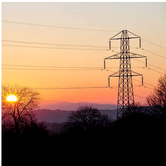
Transmission Line of the Eastern Network (Dundo - Lucapa - Saurimo - Luena) and Associated Substations | 220 kV | Angola Client: MINEA Basic Design and Tender Documents; Environmental and Social Impact Assessment: 2012/2015
