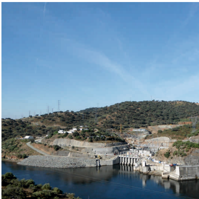
Very High Voltage Line between Alqueva II and Alqueva Substation | 400 kV Portugal Client: EDP – Electricidade de Portugal Environmental Constraints Study and Environmental Impact Assessment: 2007/2008
