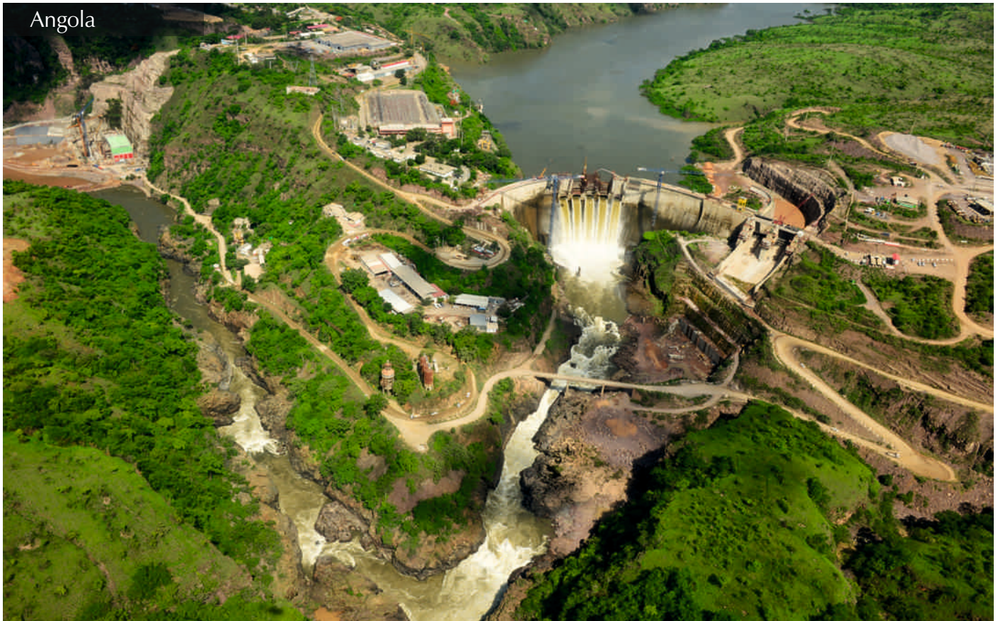
Cambambe Hydropower Development – Powerplant II. Overall Coordination and Construction works Supervision. Environmental Follow-up of the Construction Works. GAMEK – Gabinete de Aproveitamento do Médio Kwanza | Angola | 2014/15
