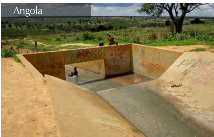
Luena Water Supply System. Design Review and Supervision of the Construction works | MINEA / DNAAS | Angola | 2013
