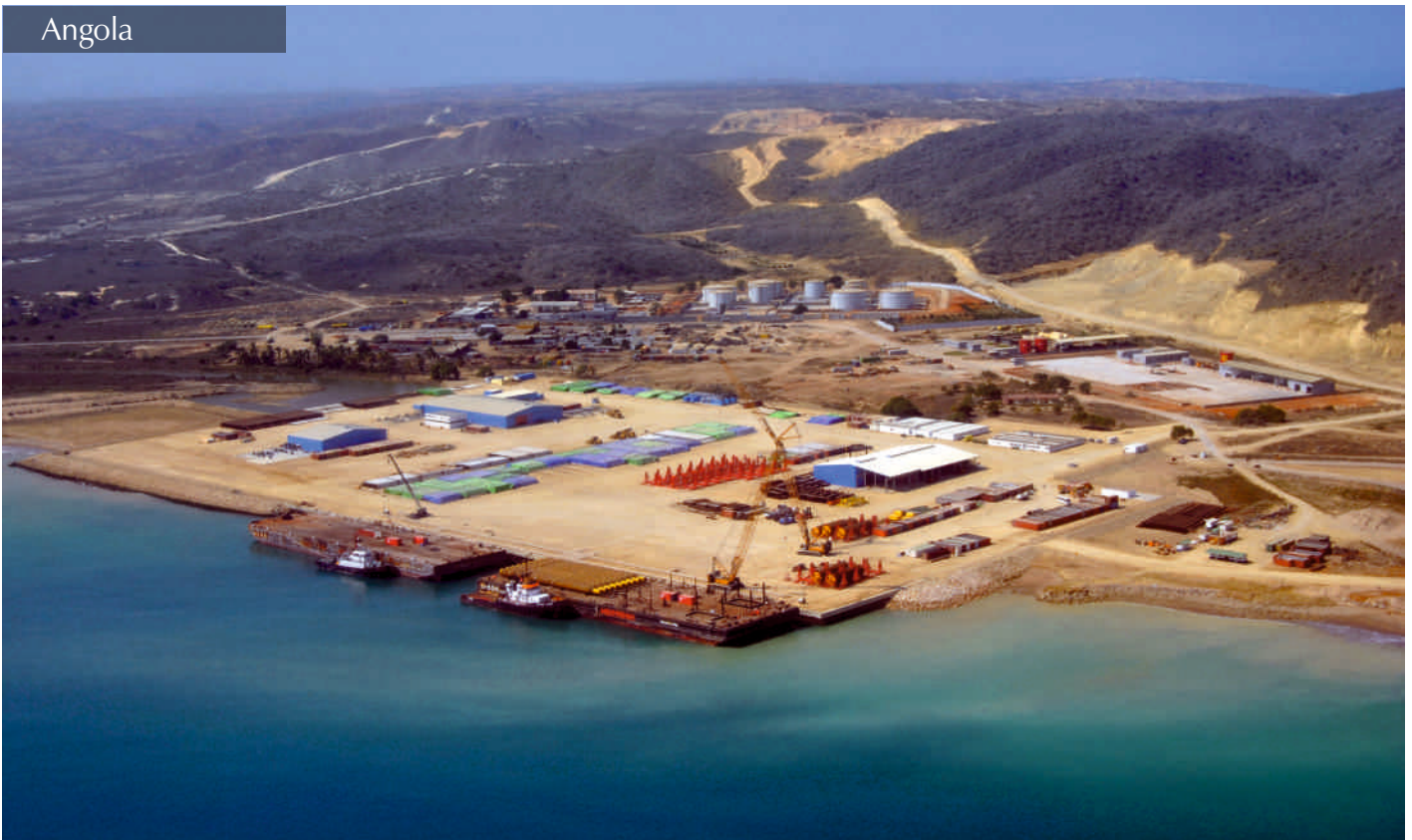
Environmental Audit of the PAENAL Facilities | PAENAL - Porto Amboim Estaleiros Navais, Lda | Angola | 2014
