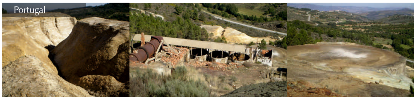
Portugal Environmental Recovery of the Former Santo António de Penedono Mining Area | EDM – Empresa de Desenvolvimento Mineiro | Portugal | 2006/07
