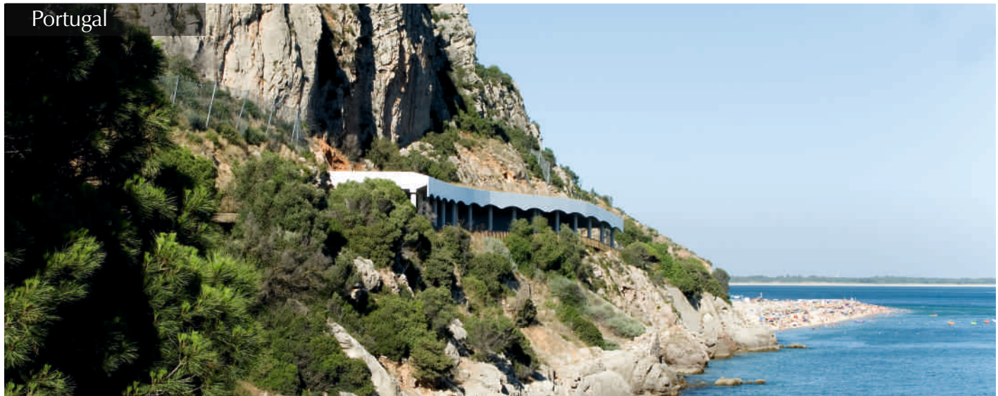
Portugal Slope treatment and Stability of National Road EN 379-1 between Outão and Portinho da Arrábida | EP – Estradas de Portugal, EPE Portugal | 2005/06
