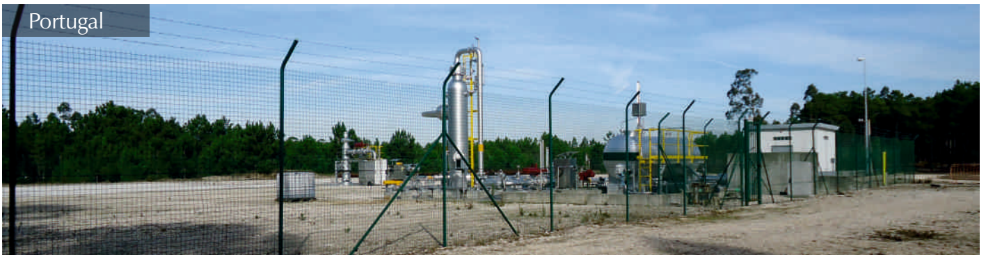
Project for Construction of Three Cavities for Natural Gas Storage at Carriço | REN / TRANSGÁS | Portugal | 2011/12
