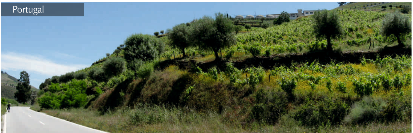
Landscaping Design of National Road EN222, between km 131+500 and km 152+000 – Stabilization of Slopes between Torrão (in the vicinities of Régua) and the “Bateiras” Bridge EP, Estradas de Portugal, S.A. | Portugal | 2010
